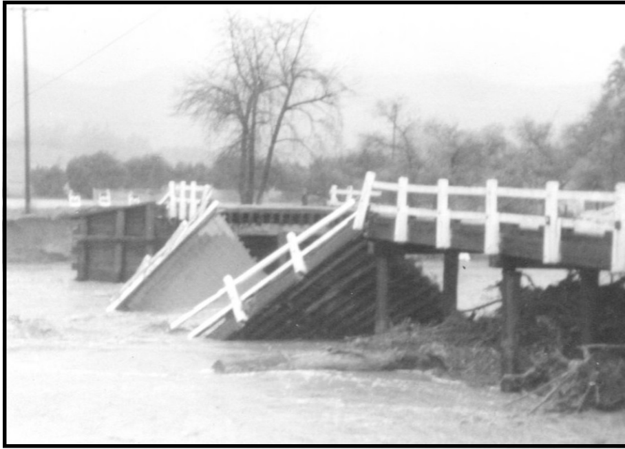
The B Street Bridge collapsed during the Flood of 1978
