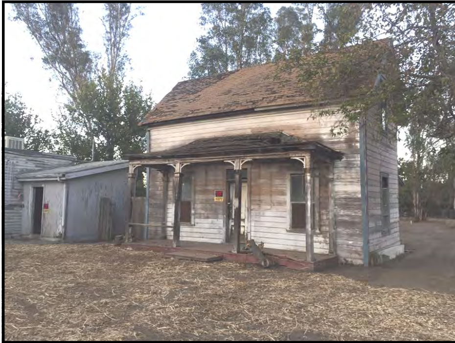
The Lakeman House, October 13, 2017
