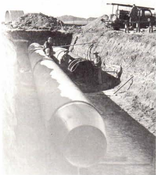
Above are the two pipes that will carry the water from the valves into the channel and eventually the lake. Left to right is Jack Carroll, Chet Ryals and Toby Taylor, carpenter foreman. All of the men in the photos are employed by the Metropolitan Water District.
