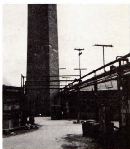
Gas pipes which deliver the gas to some 20 kilns.
