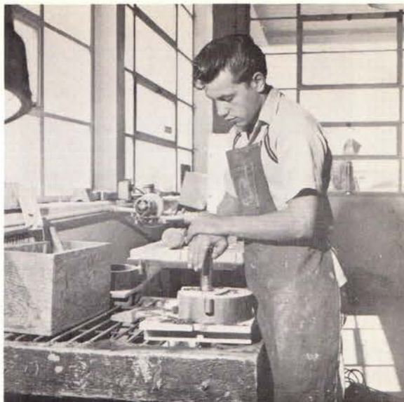
Preparing to cast, George Suniga forces sand into a mold.
